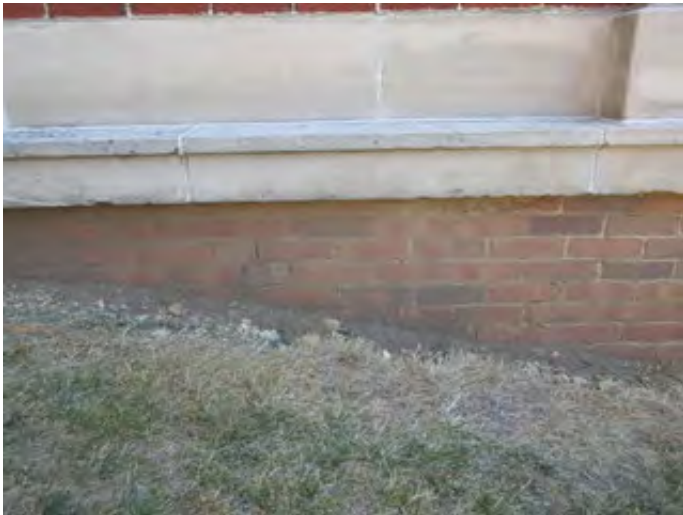
Typical Masonry Foundation of the Original Construction
