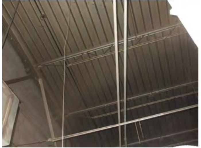
Typical Roof Structure of the 1951 Pre-Kindergarten Annex
