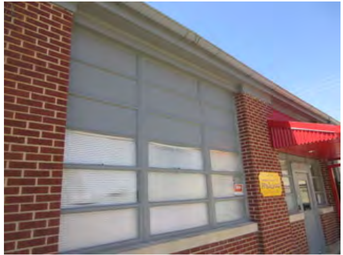
Typical Steel Windows of the 1951 Annex
