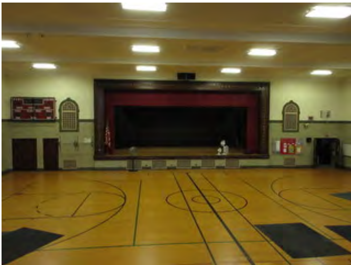
Gymnasium Fluorescent Lighting Fixtures
