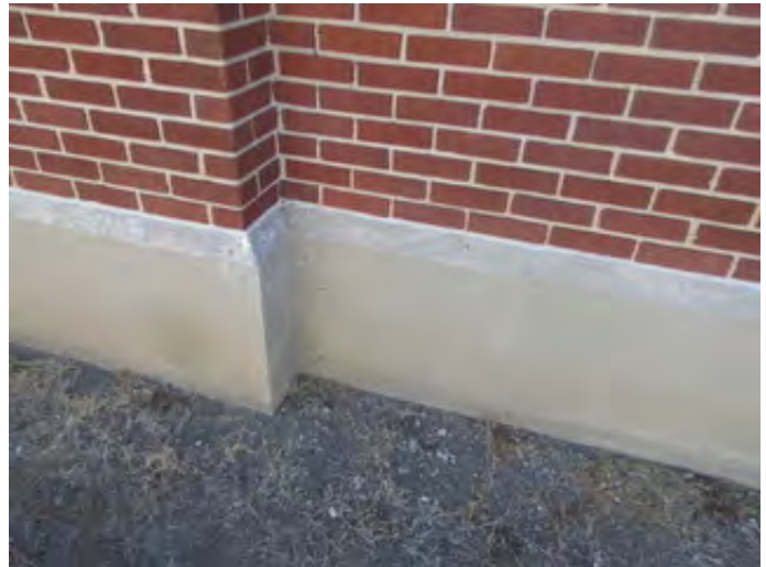
Typical Concrete Foundation of the 1930 Gymnasium Addition
