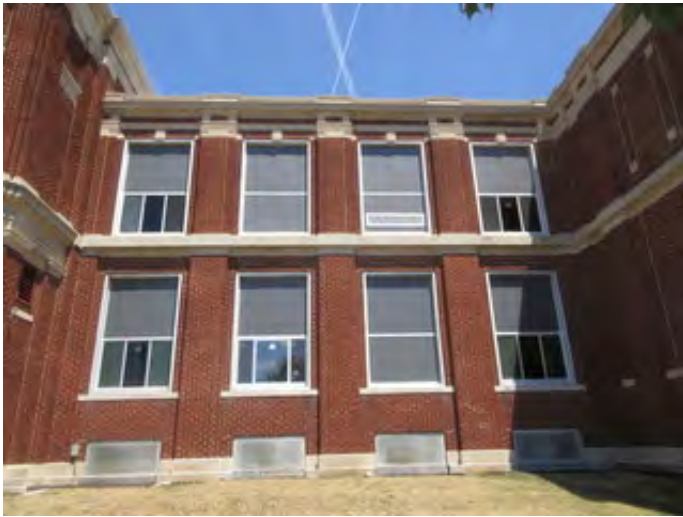
Typical Aluminum Windows of the Original Construction
