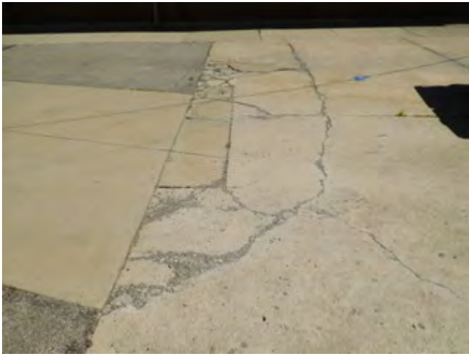
Concrete Dumpster Pad
