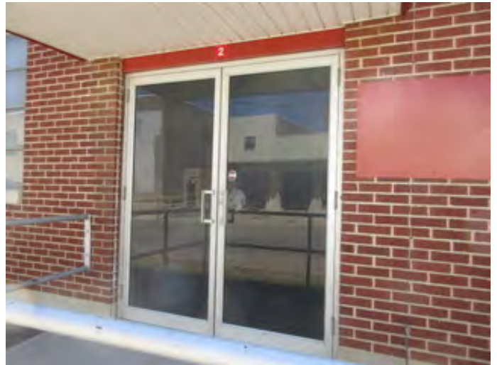
North Entrance Doors of the 1951 Pre-Kindergarten Annex
