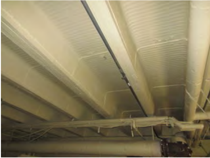
Typical Concrete Floor Structure of the 1930 Gymnasium Addition
