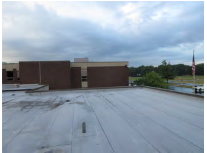
Waste Vent Piping
