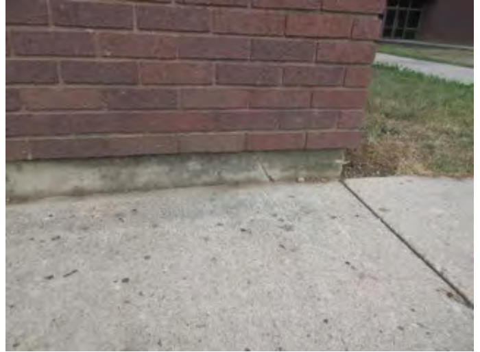
Minor Foundation Repair
