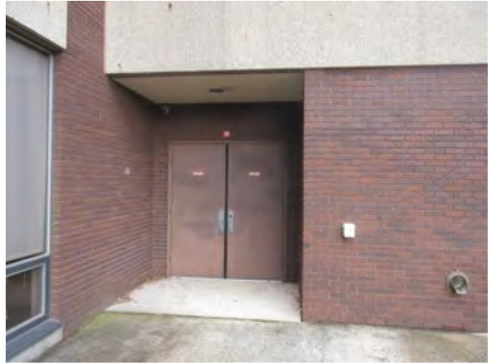
Typical Exterior Doors
