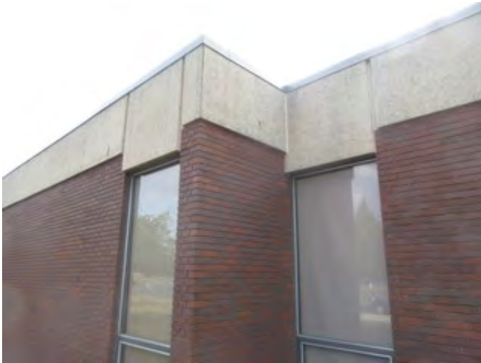
Precast Concrete Panels
