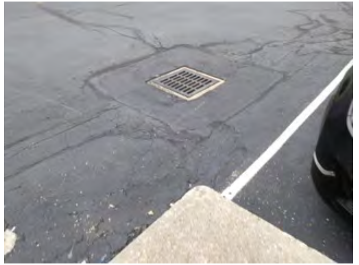
Parking Lot Catch Basin
