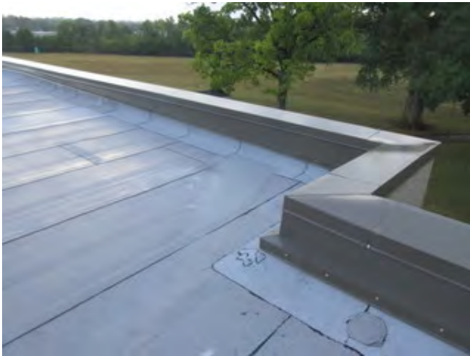
Typical Coping and Roofing
