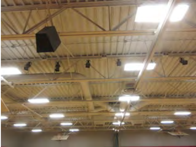
Steel Joist Roof Structure
