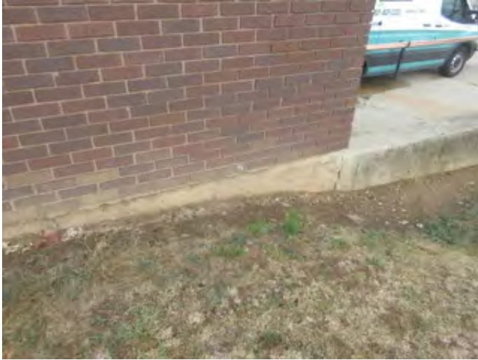
Typical Concrete Foundation
