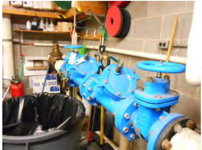
Reduced Pressure Backflow Preventer
