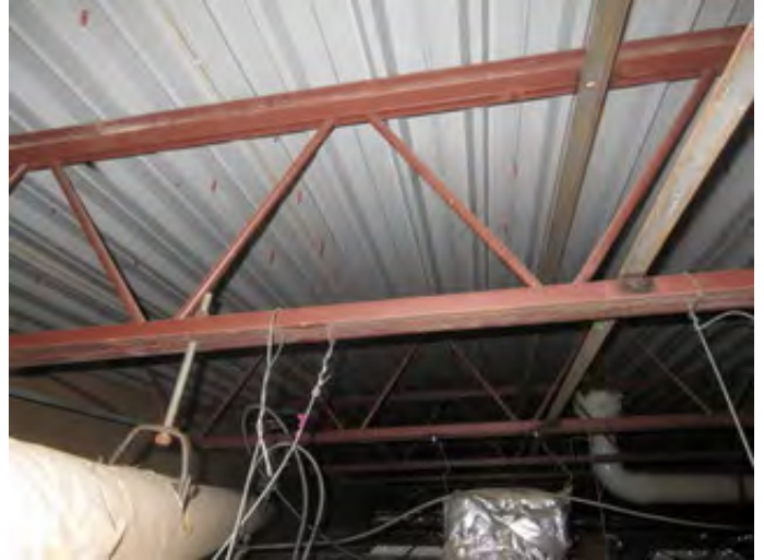
Steel Joist Roof Structure
