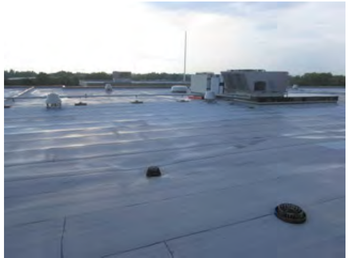
Typical Primary and Overflow Drains
