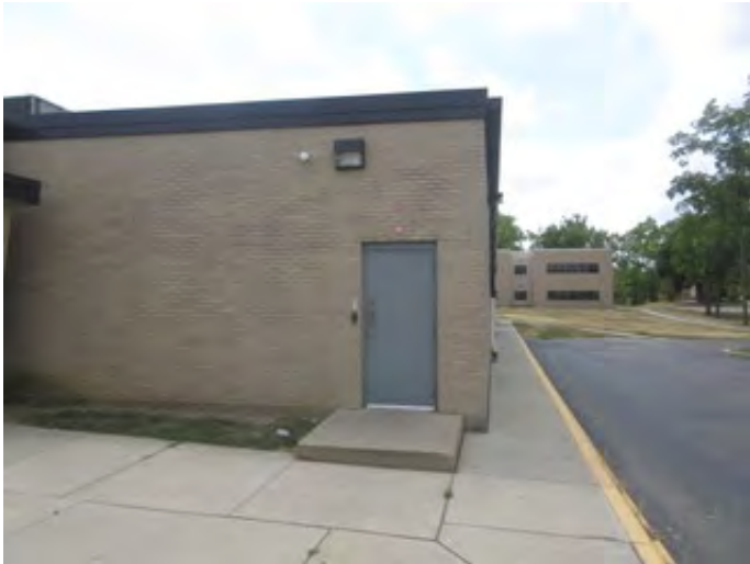
Typical Exterior Door
