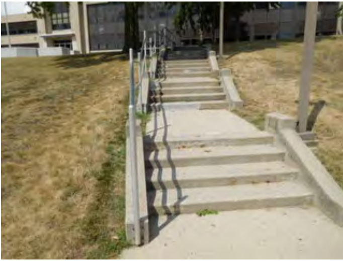
Concrete Steps, Sidewalk, and Handrails
