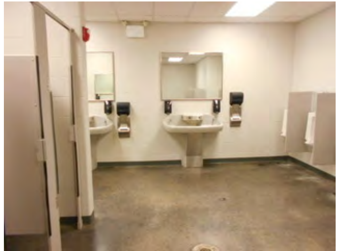
Large Group Restroom-Boys-2006 Addition
