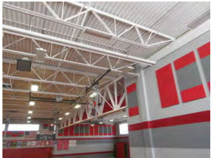
Steel Structure of the 2006 Gymnasium & Classroom Addition
