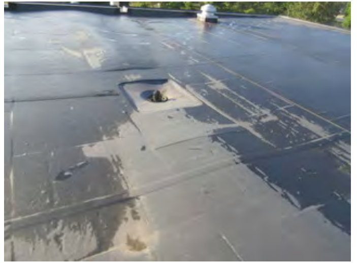
Typical EPDM Roofing
