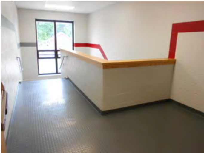
Compliant Enclosed Stair Tower-2006 Addition
