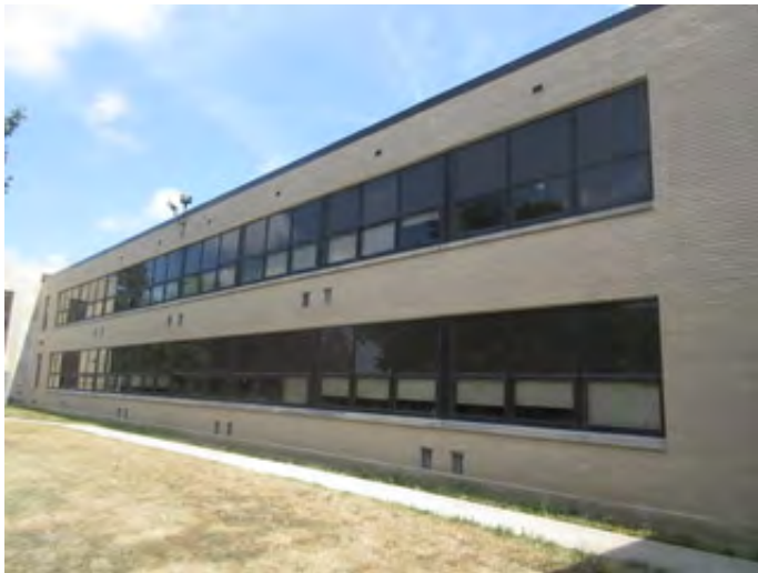
Typical Aluminum Windows of the Original Construction
