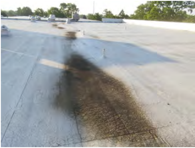
Typical Tremco Roofing
