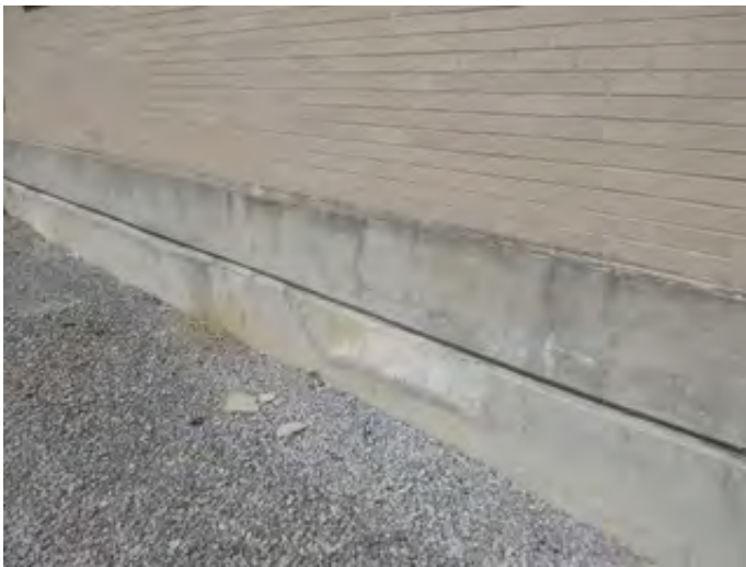
Minor Foundation Repair
