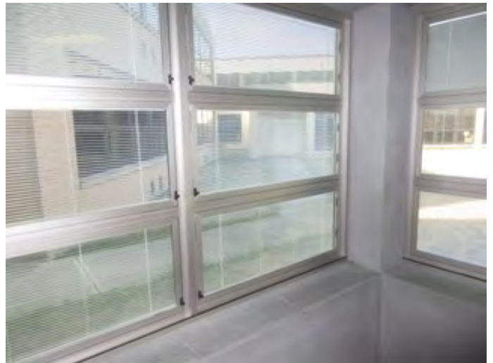
Typical Windows with Integral Blinds in the 2006 Gymnasium & Classroom Addition
