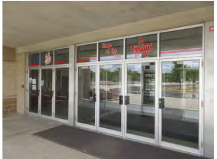
Entrance Doors of the Original Construction
