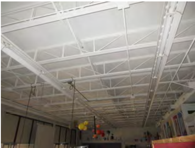
Steel Joist Structure of the Original Construction
