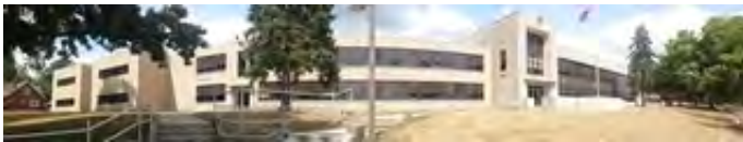
South elevation photo:
