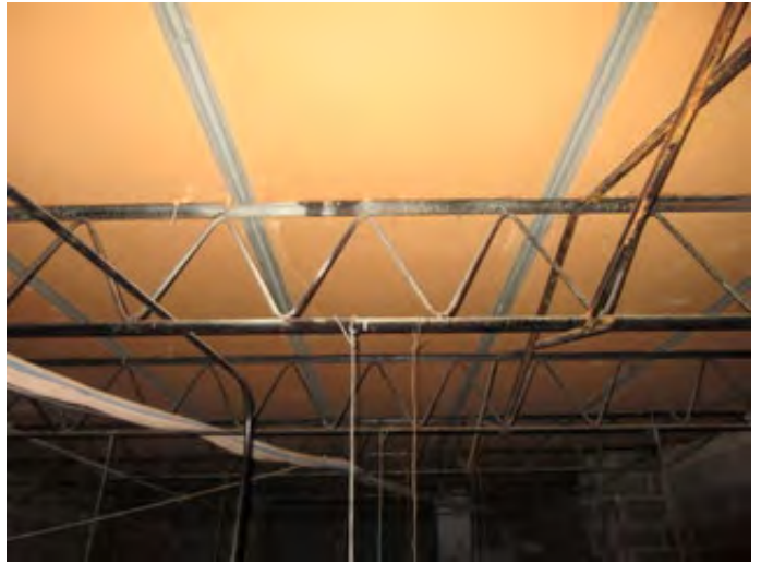
Typical Roof Structure of the Original Construction
