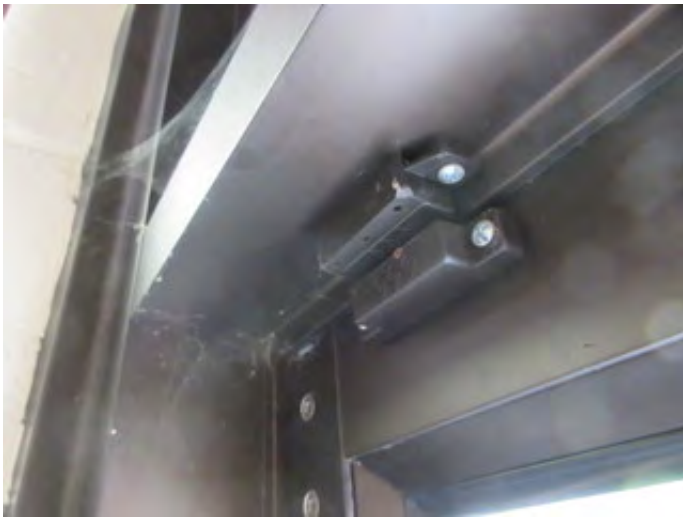
Security System Door Contacts
