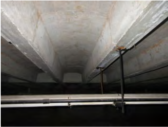
Typical First Floor Framing of the Original Construction
