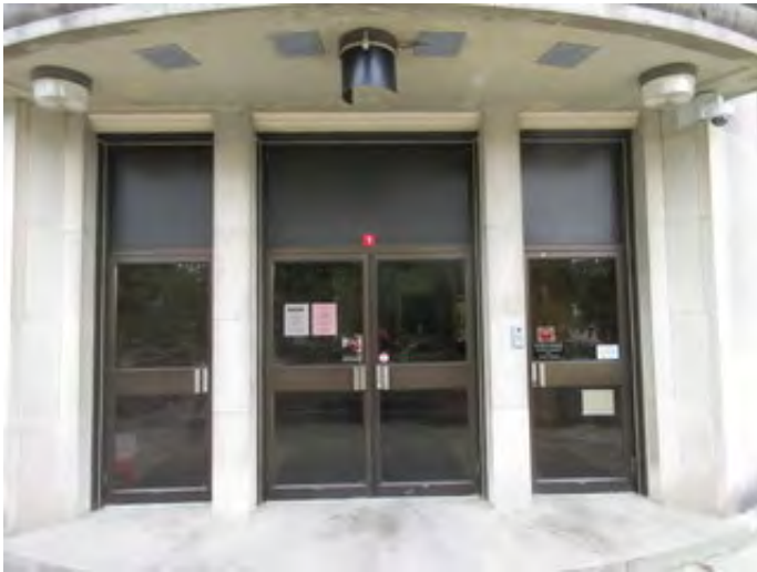
Main Entrance Doors
