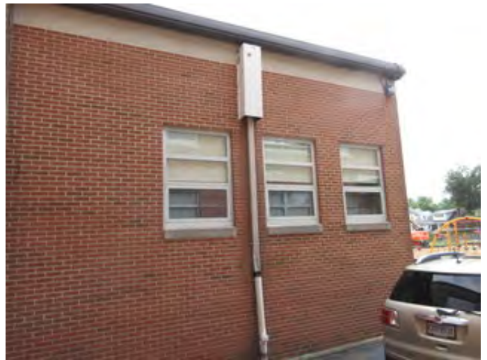
Downspout of 1974 Kitchen Addition
