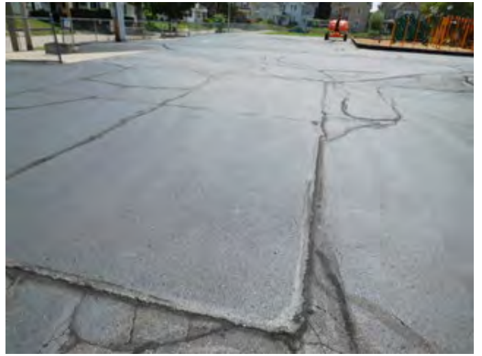
Typical Condition of Asphalt
