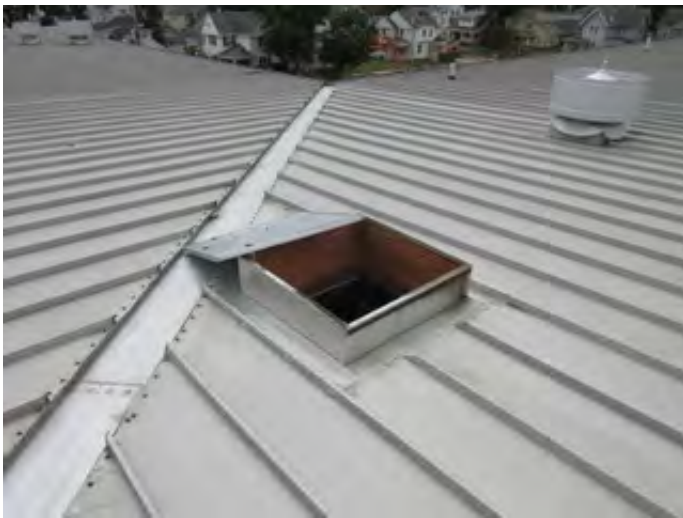
Access Hatch & Standing Seam Metal Roof
