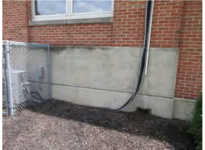
Minor Foundation Repair
