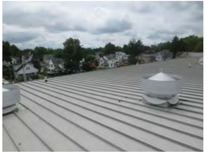
Waste Vent Piping
