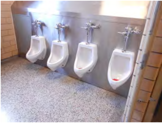
Urinals at ADA Compliant Height
