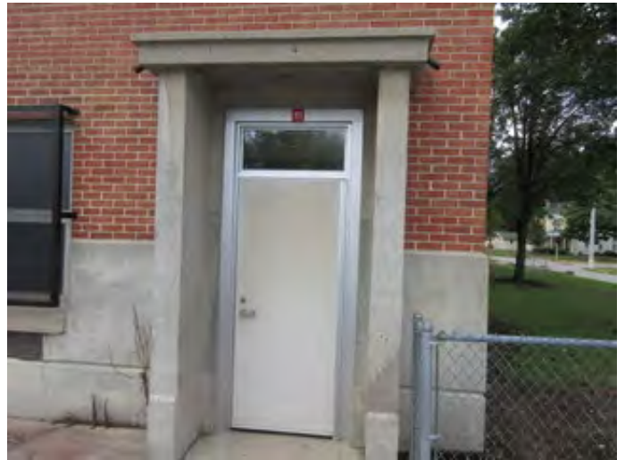
Typical Exterior Doors
