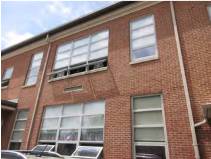
Typical Aluminum Windows of the Original Construction
