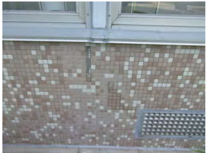
Mosaic Ceramic Tile Repairs
