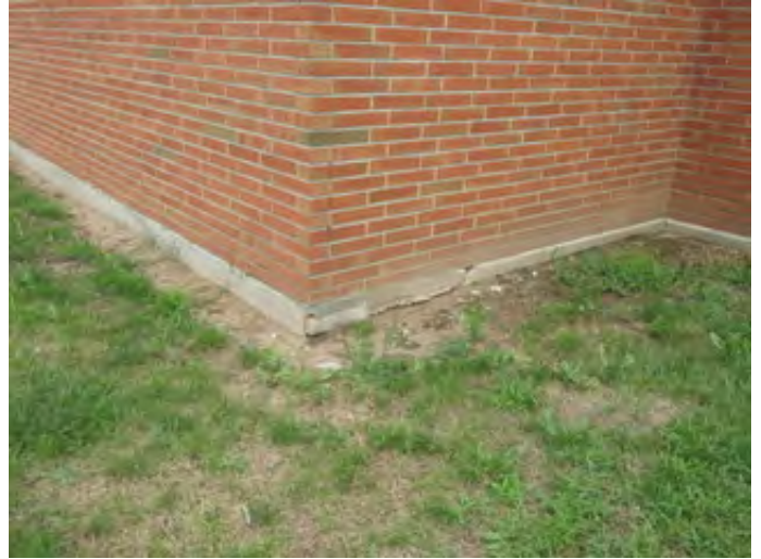
Minor Foundation Repair
