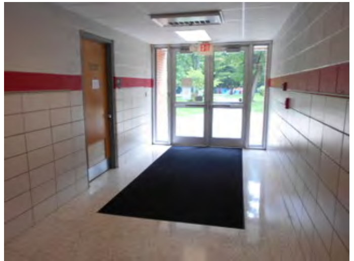
Compliant Exit Corridor
