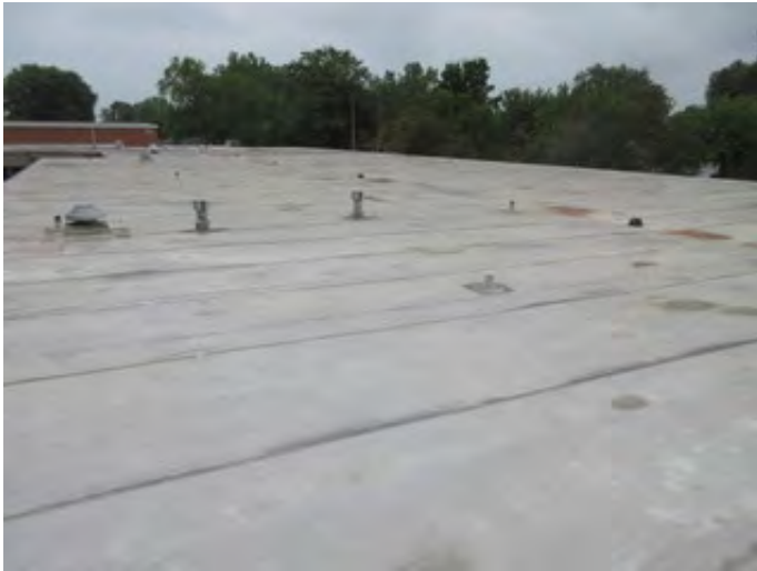
Typical PVC Roofing
