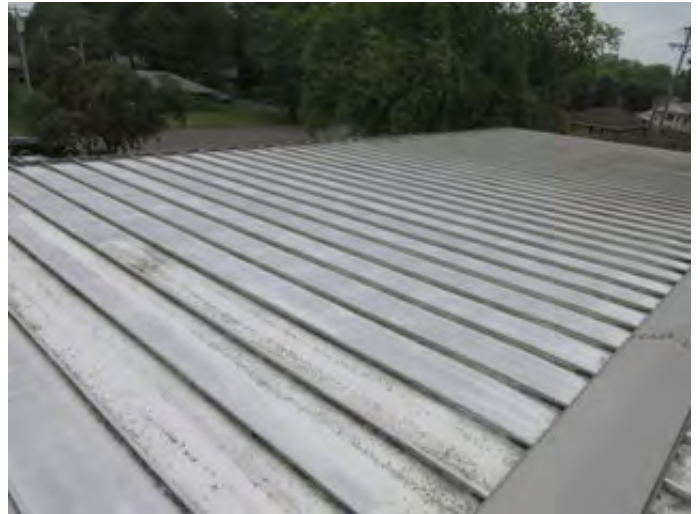
Standing Seam Metal Roofing Over the Stage and Multi-Purpose Room
