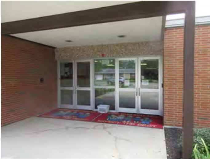
Main Entrance Doors
