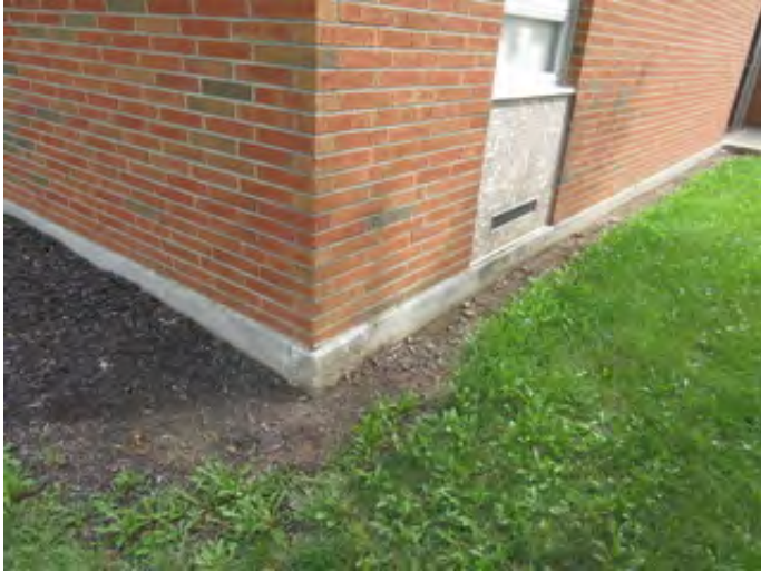
Typical Concrete Foundation
