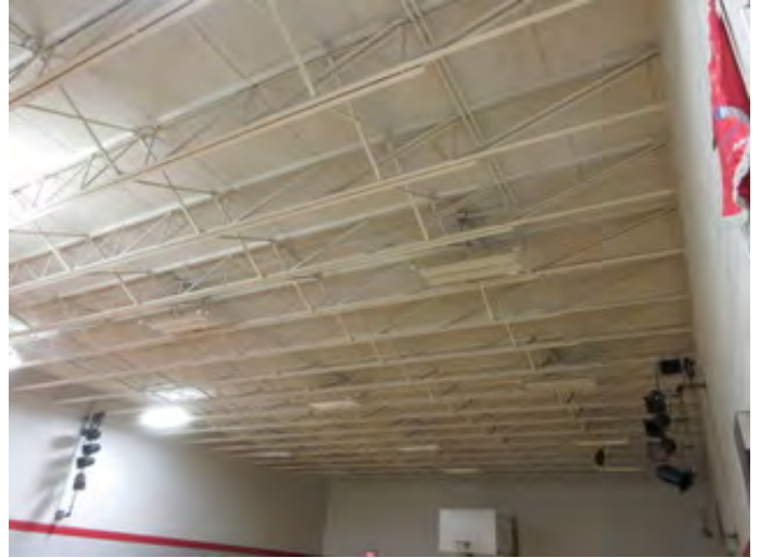
Typical Tectum Deck Roof Structure
