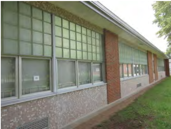
Typical Windows of the Original Construction
