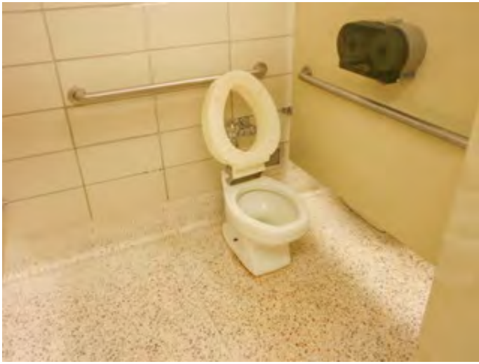
ADA Compliant Toilet Stall
