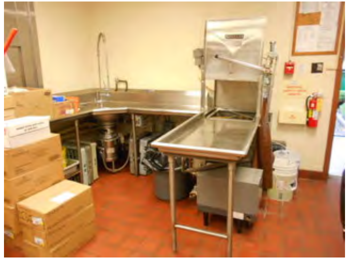
Commercial Dishwasher with Heat Booster
