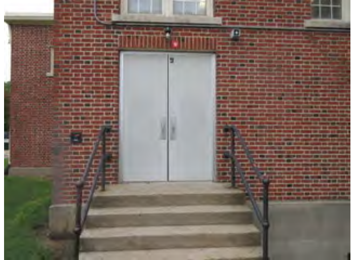
Typical Exterior Doors
