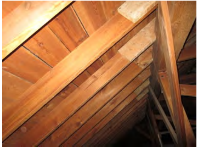
Wood Rafters and Decking
