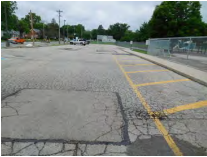
Asphalt Parking Lot Condition
