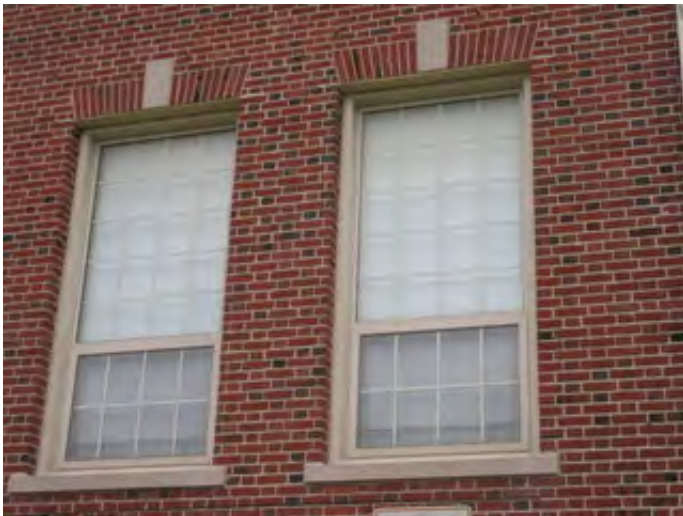
Typical Aluminum Windows of the Original Construction
