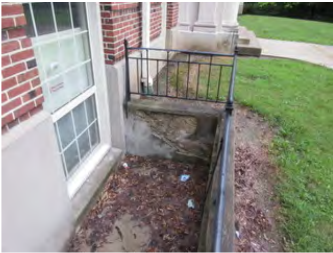
Replace Concrete Window Wells
