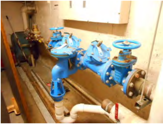
Reduced Pressure Backflow Preventer
