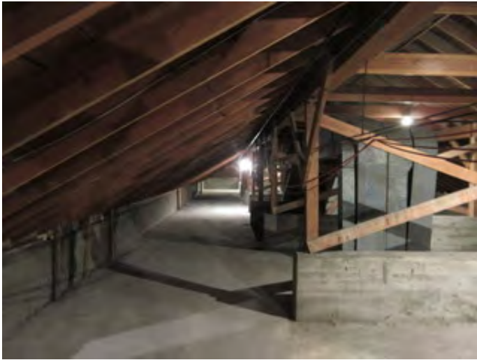
Typical Concrete Attic Floor & Wood Rafters
