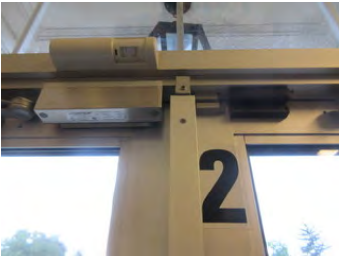
Security System Door Contacts
