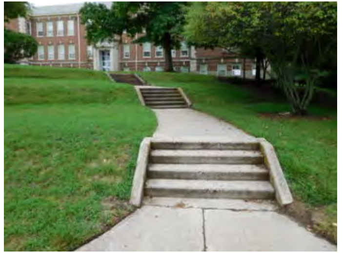
Exterior Concrete Steps and Sidewalk
