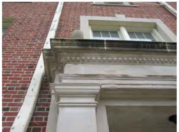
Typical Stone Repairs
