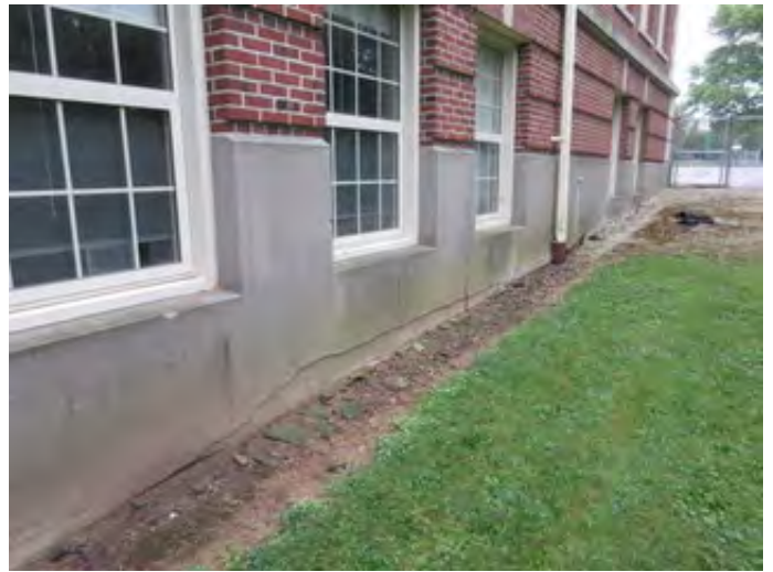
Minor Foundation Repair
