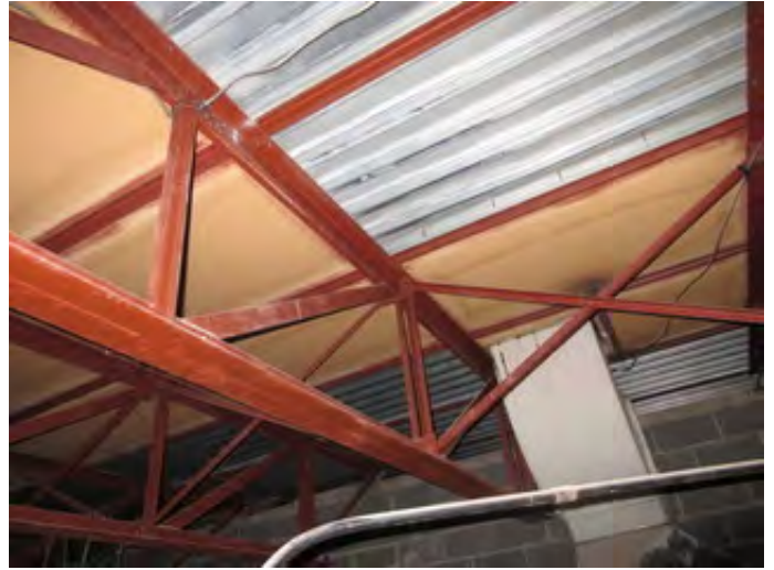
Combination of Gypsum and Steel Roof Deck of the Original Construction
