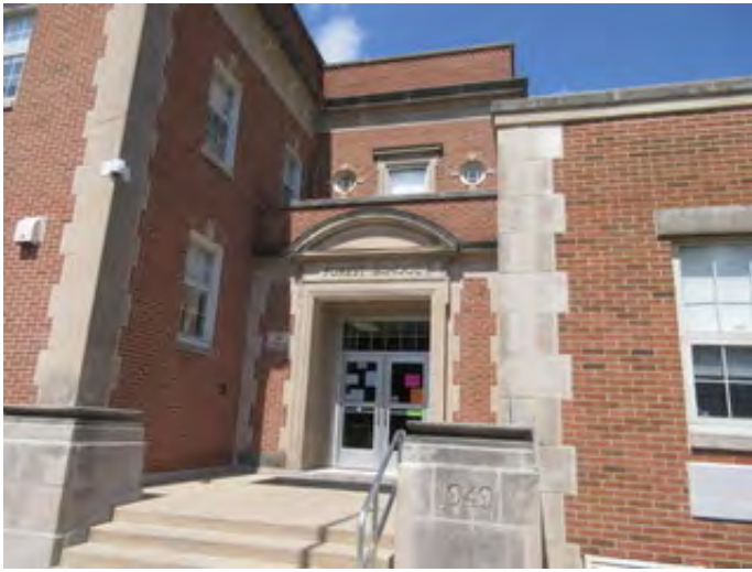
Typical Masonry and Stone Accents of the Original Construction
