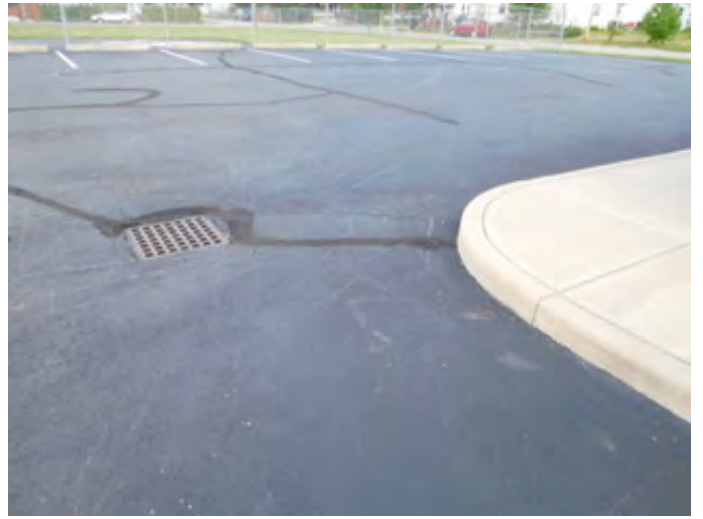
Asphalt Parking Lot and Catch Basin
