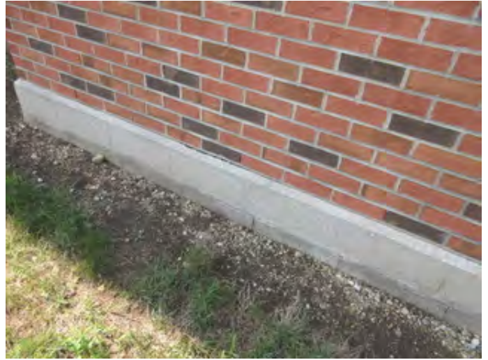
Typical Concrete Masonry Foundation of the 2006 Kindergarten Addition
