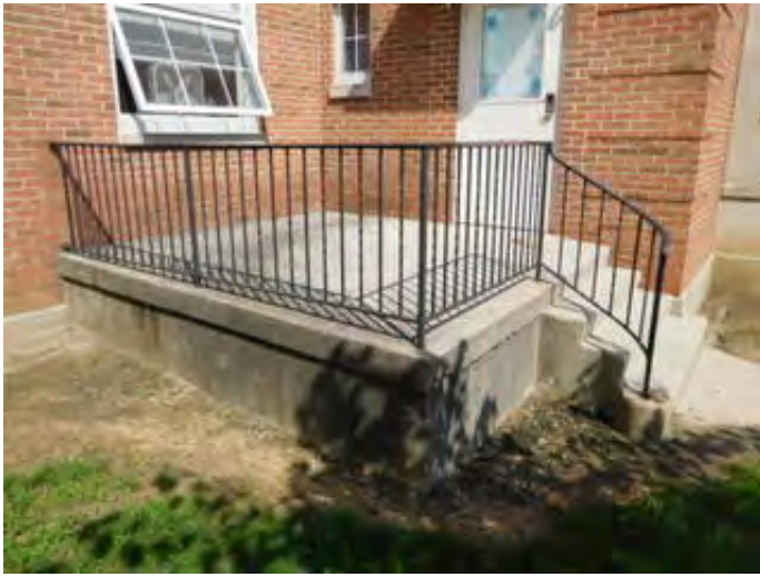
Concrete Steps and Handrail/Guardrail
