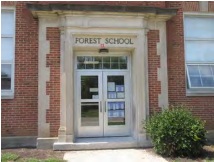
Typical Entrance Doors of the Original Construction
