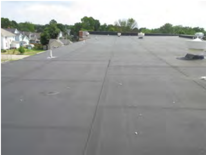
Typical EPDM Roofing of the Original Construction
