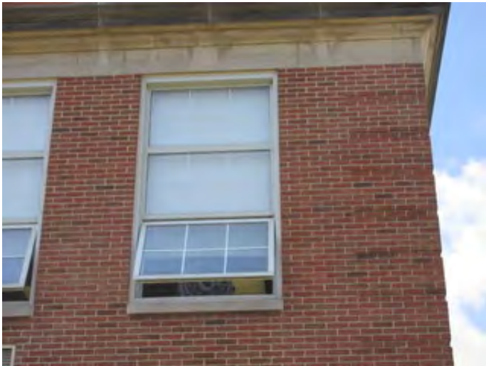
Typical Aluminum Windows of the Original Construction
