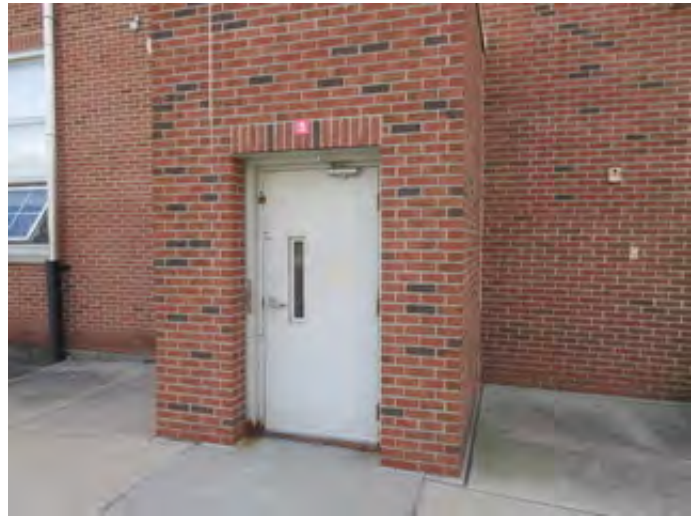
Typical Hollow Metal Exterior Door
