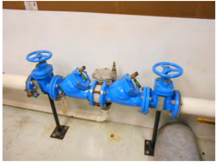
Reduced Pressure Backflow Preventer
