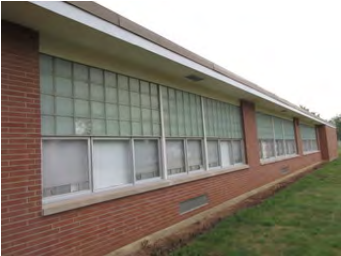
Typical Windows of the Original Construction
