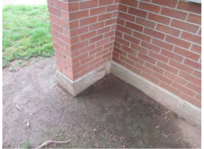
Minor Foundation Repair
