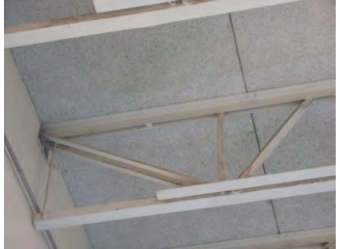
Typical Roof Structure of the Original Construction
