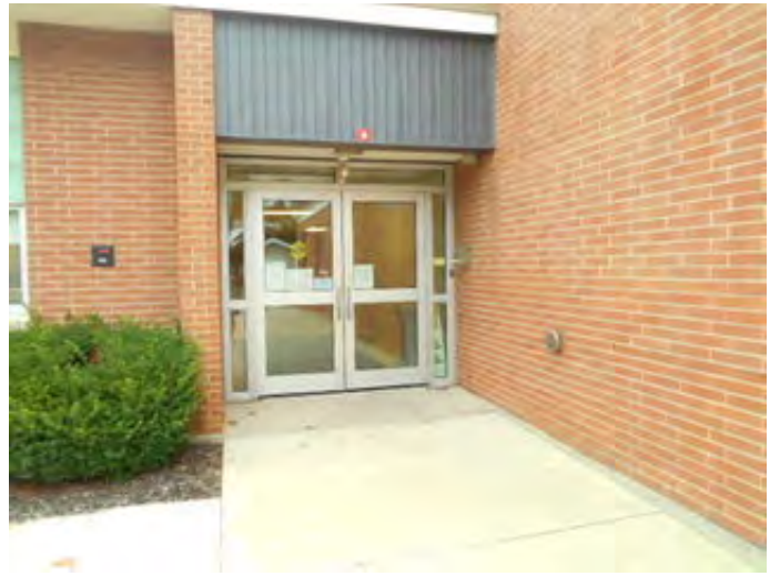
ADA Compliant Power Assisted Door
