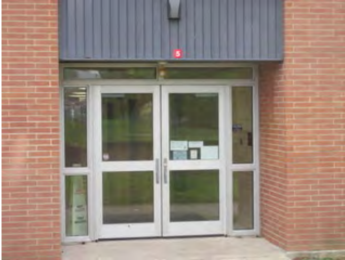
Typical Entrance Doors of the Original Construction
