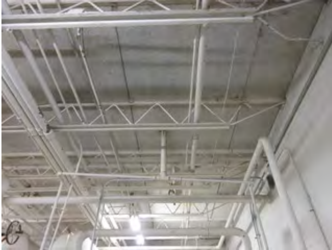
Typical Roof Structure of the Original Construction
