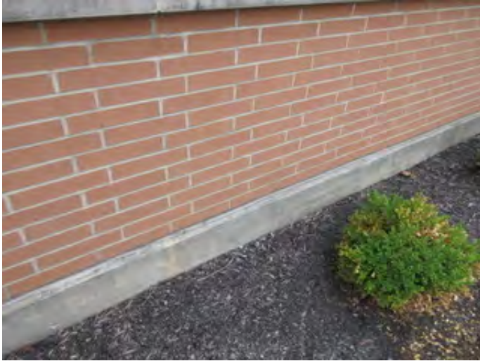
Typical Foundation of the Original Construction
