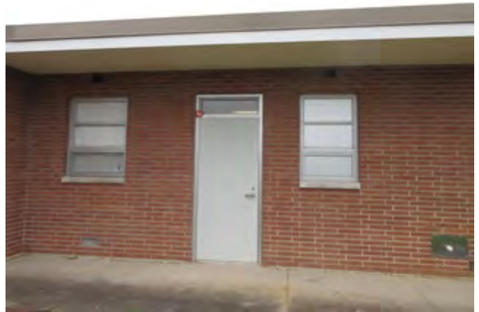
Typical Exterior Door of the Original Construction
