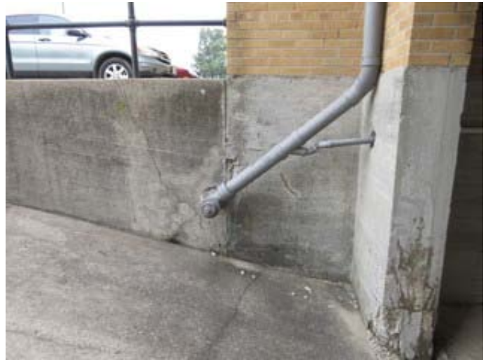
Foundation Repair at 1939 Gymnasium Addition
