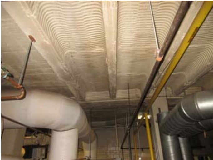
Typical Concrete Floor Structure of the 1939 Gymnasium Addition
