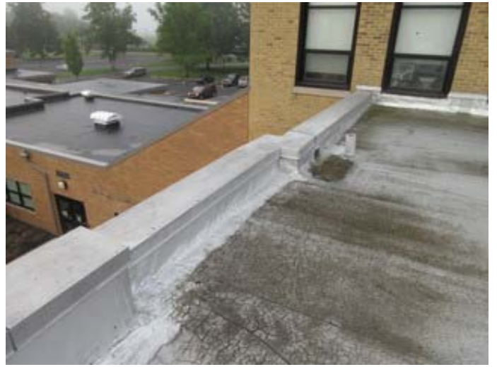
Tremco Roofing and Coping of the 1939 Gymnasium Addition
