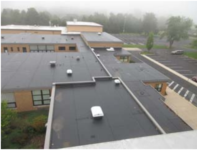
EPDM and TPO Membrane Roofs
