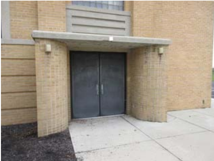
Fiber-Reinforced Plastic Doors of the 1939 Gymnasium Addition
