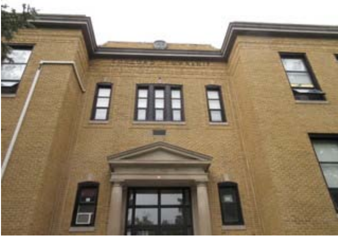
Masonry of the Original Construction
