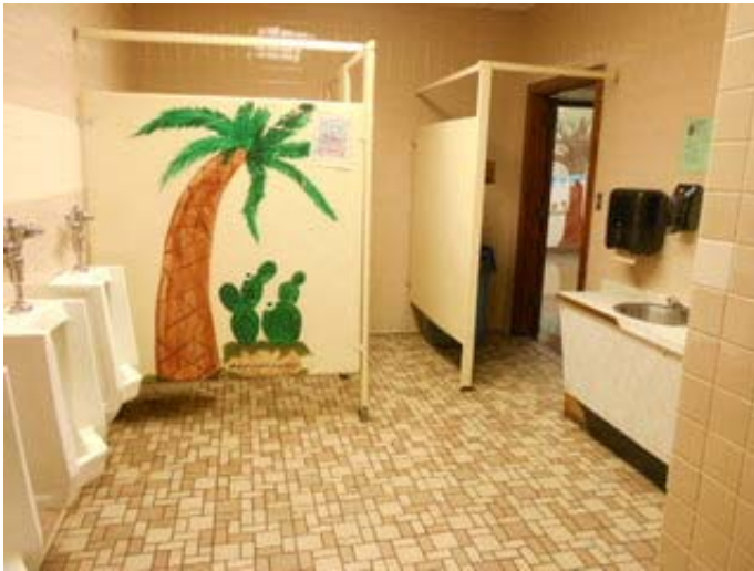
Large Group Restroom-Boys-1919 Original Construction
