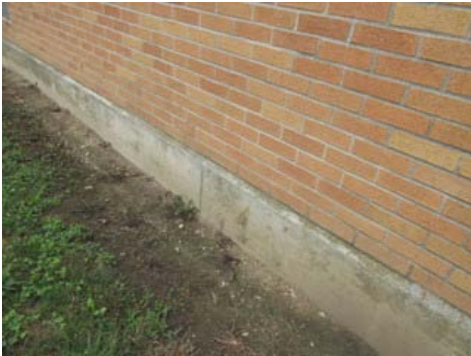
Typical Concrete Foundation
