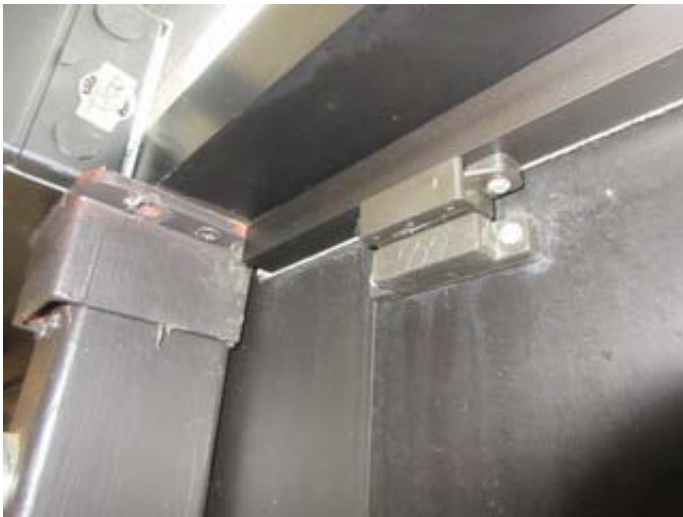
Security System Door Contacts
