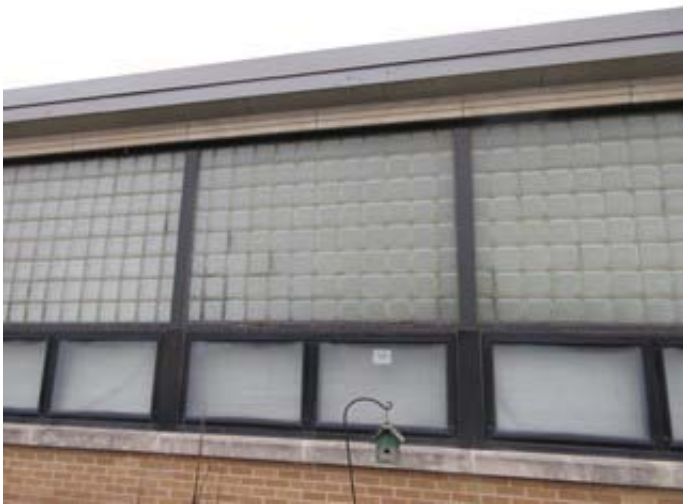
Typical Aluminum and Glass Block Windows of the 1952 Classroom Addition
