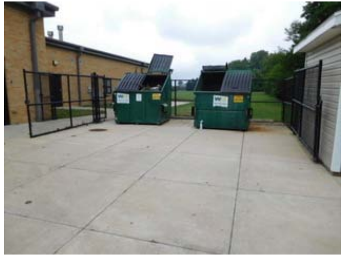
Concrete Dumpster Pad
