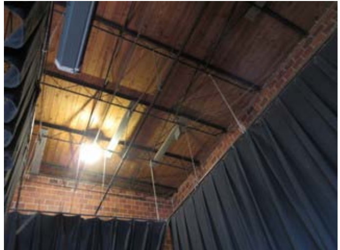
Wood Roof Deck of the 1939 Gymnasium Addition
