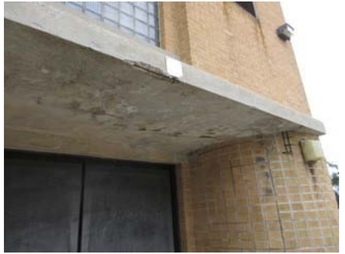
Concrete Repair of the 1939 Gymnasium Addition
