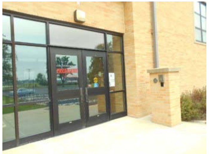
ADA Compliant Power Assisted Door
