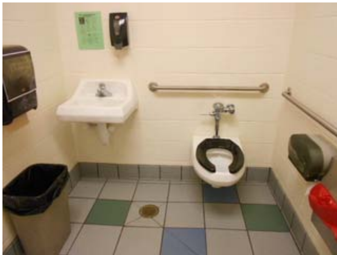
ADA Compliant Unisex Restroom
